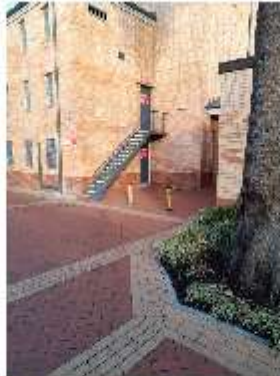
Stage door and Dressing Room access
