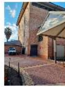
Loading Dock. Overhead obstruction
