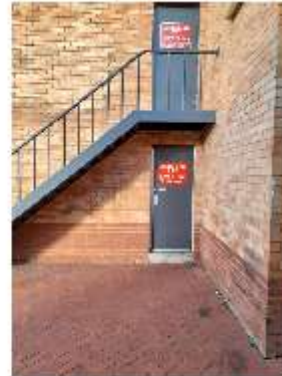
Stage door and Dressing Room access
